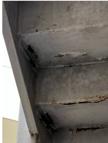
Image 8: West- Flaking of paint and corroded welds at 3 rd level steps/stringer
