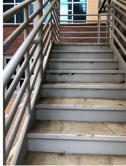
Image 14: East- Stage 4 corrosion present at steps
