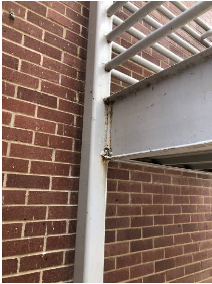
Image 17: East- Weld conditions
