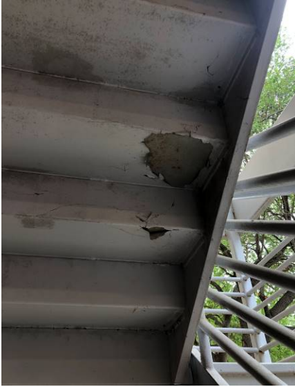
Image 5: West- Flaking of paint present at steps
