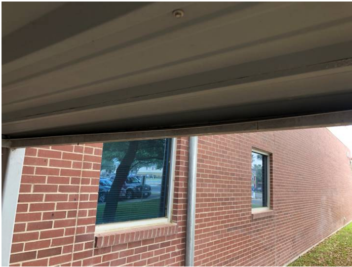
Image 3: West-Deflection at perimeter deck angles.
