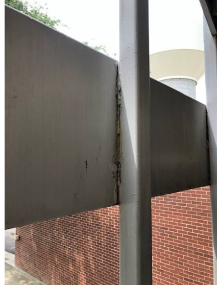
Image 6: West-Weld corrosion at 24" deep channel
