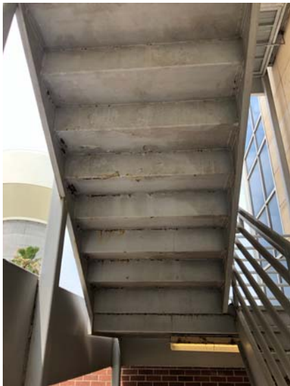
Image 7: West- Corroded welds at 3 rd level steps.
