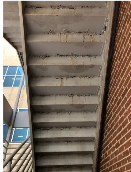
Image 18: East-Weld conditions
