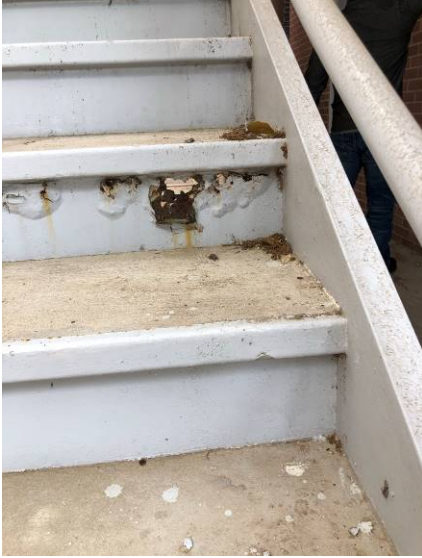
Image 13: East-Stage 4 corrosion present at steps
