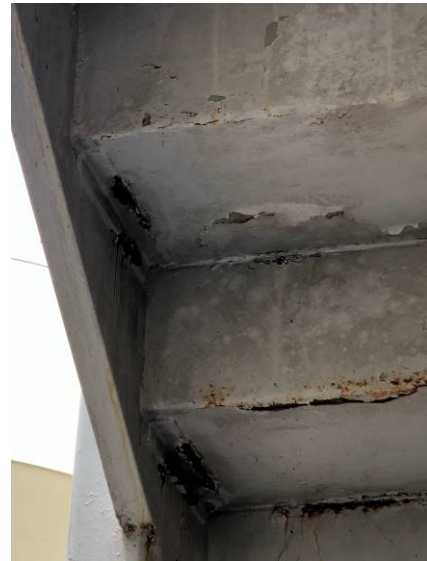
Image 8: West- Flaking of paint and corroded welds at 3 rd level steps/stringer
