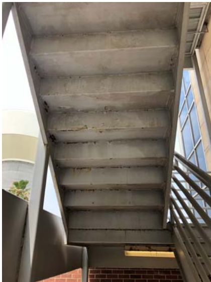
Image 7: West- Corroded welds at 3 rd level steps.
