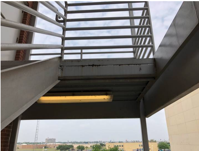
Image 19: East- Weld conditions
