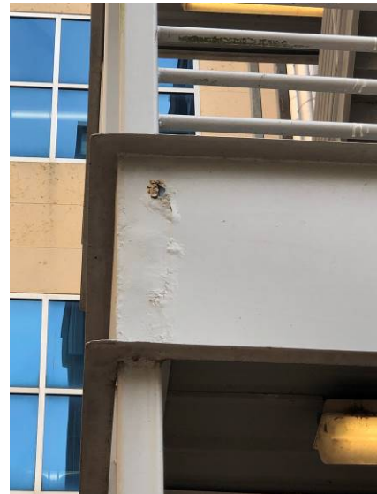
Image 20: East-Flacking of paint present
