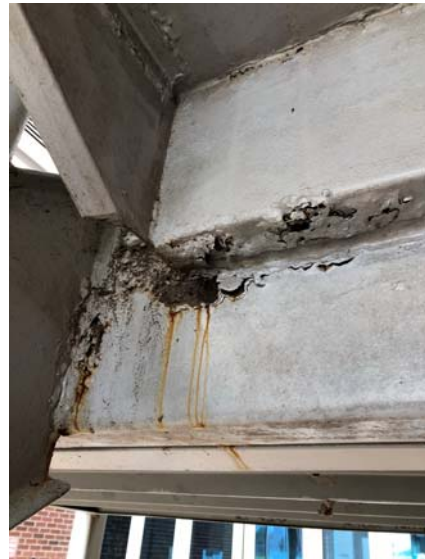
Image 16: East-Weld conditions
