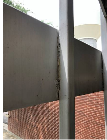
Image 6: West-Weld corrosion at 24" deep channel
