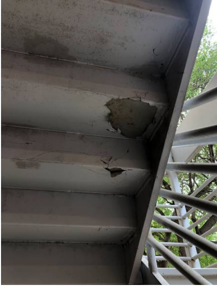
Image 5: West- Flaking of paint present at steps
