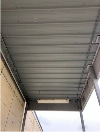
Image 9: West Flacking of paint on Roof structure
