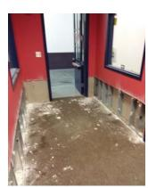
June 23, 2018 - FOM began the process of making 2 to 4 foot flood cuts in the Student Success Center, Open Computer Lab, Instructional Computer Lab, and Offices adjacent to the Student Success Center. Also, removed all baseboards throughout the building and will remove carpenting the next day.
